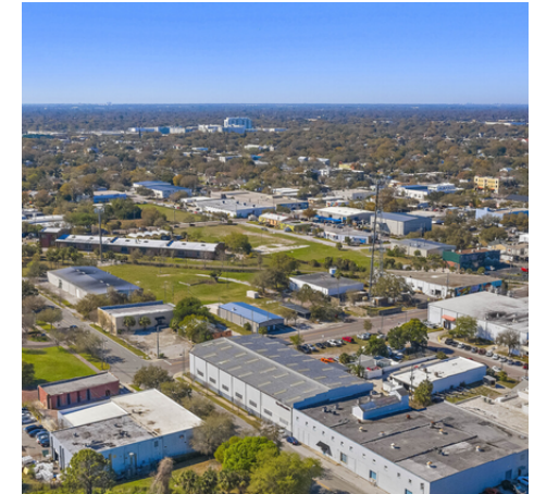
Aerial view looking northwest
