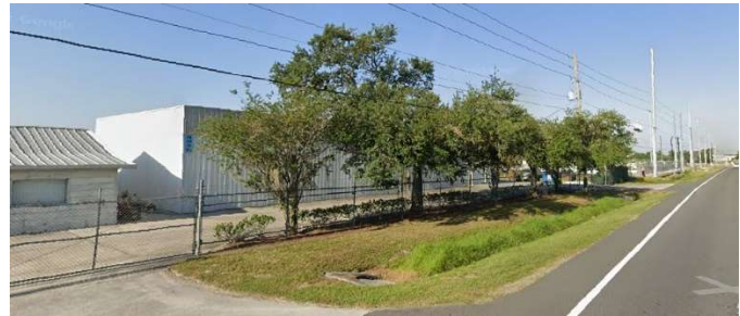
Front view – Looking west along Drane Field Road
