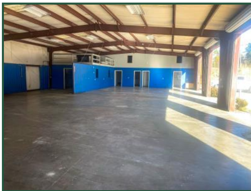
Interior, Towards Mezzanine
