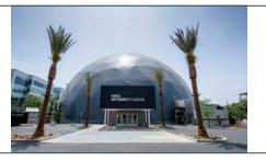
Located on Empire Avenue, the new Madison Square Garden (MSG) media services facility is a spherical geodesic 95-foot high dome with approximately 28,664 square feet of floor area on an approximate 1.95-acre vacant site. It is the prototype facility for MSG Entertainment's creative teams to develop and edit content prior to its ultimate use in Las Vegas productions.
