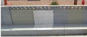
EXISTING NORTH BLOCK WALL TO BE DEMOLISHED 3'-6" HIGH
