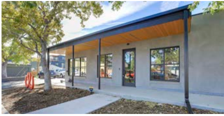
SUBJECT PROPERTY 1930 W 41st Ave., Denver, CO
