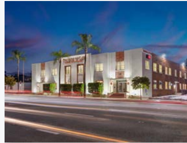
220 N GLENDALE AVE., GLENDALE, CA 91206
