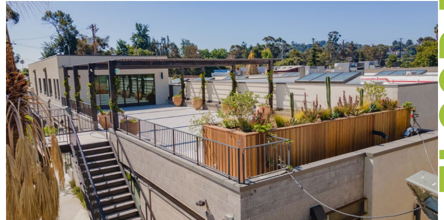
C— BUILDING B1 OUTDOOR ROOF DECK
