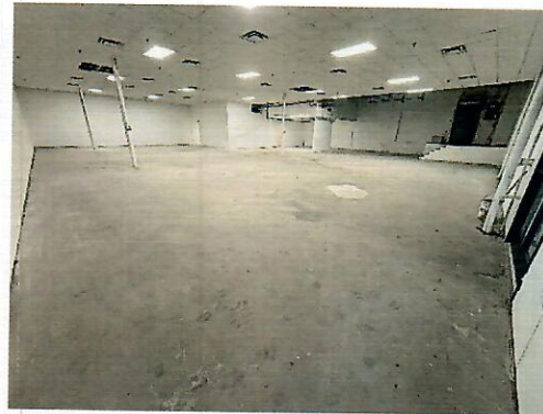
Wide open space with bathrooms in rear
