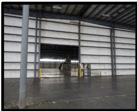
Large Forklift Passage Doors
