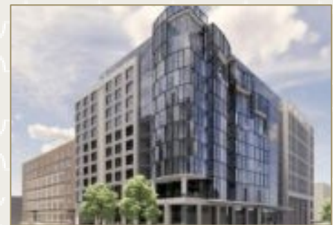
Autograph Collection & Residence Inn Hotels 350 Rooms
