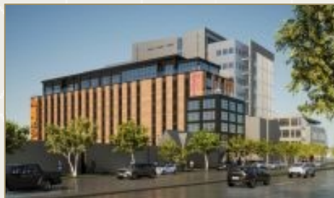
MOXY Hotel Under Construction 156 Rooms
