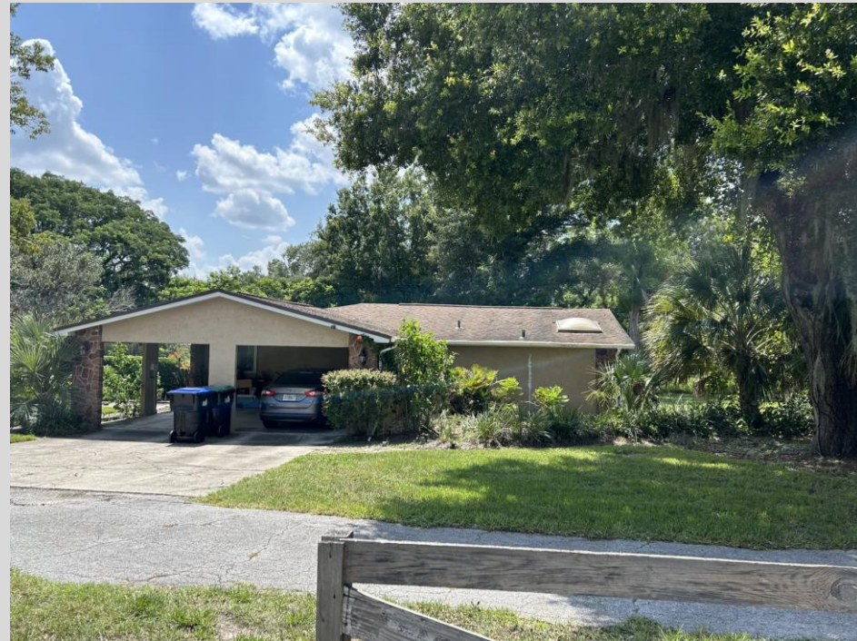
View of existing residence from the east
