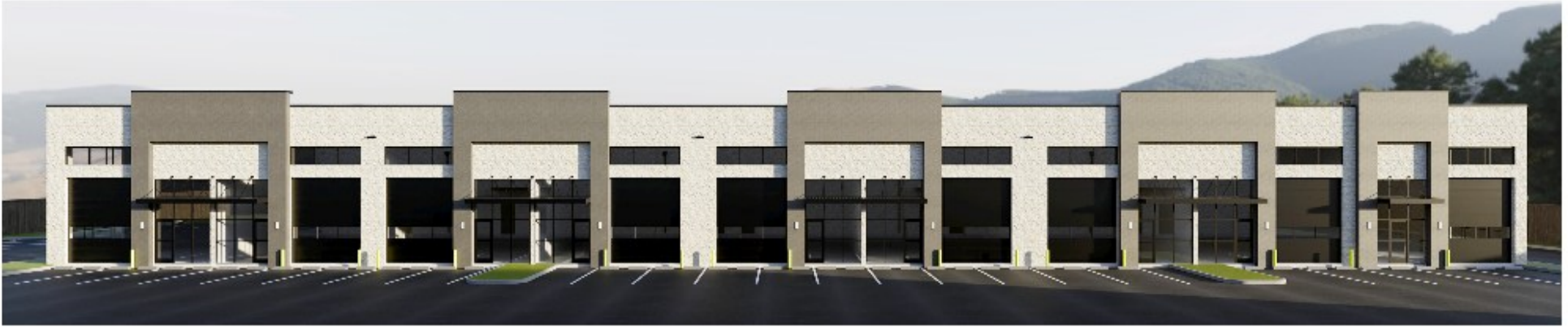
FLEX BUILDING FRONT VIEW
