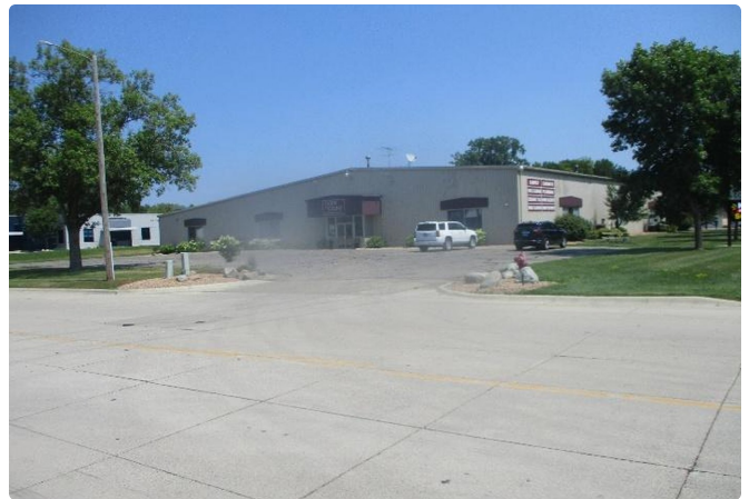
WEST ELEVATION FROM 19TH STREET NW
