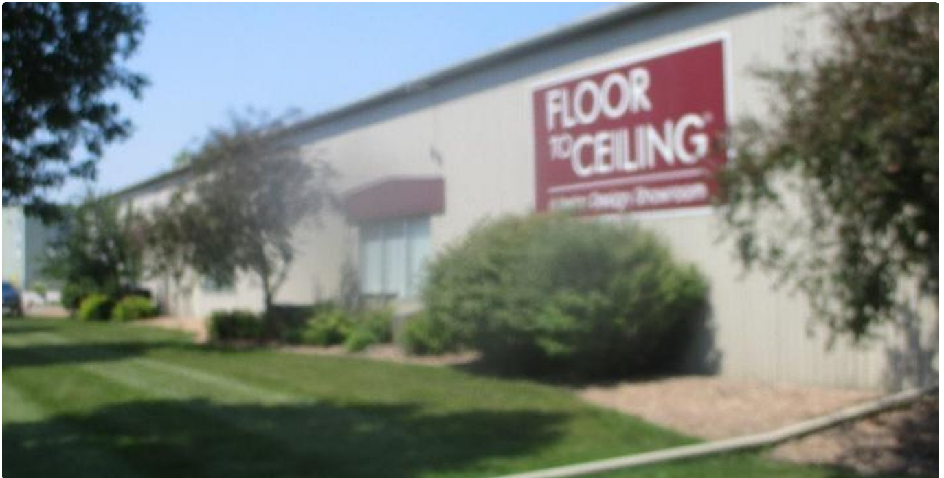
SOUTHWEST CORNER — BUILDING SIGNAGE FACING U.S. HIGHWAY 12
