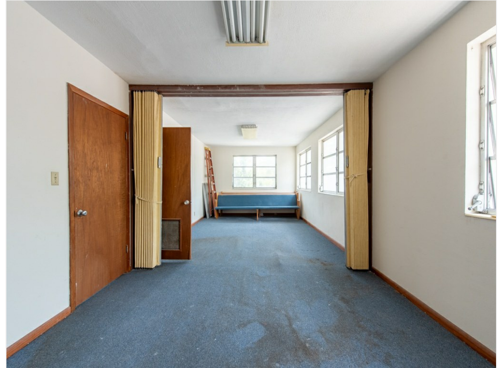
2nd Floor Office
