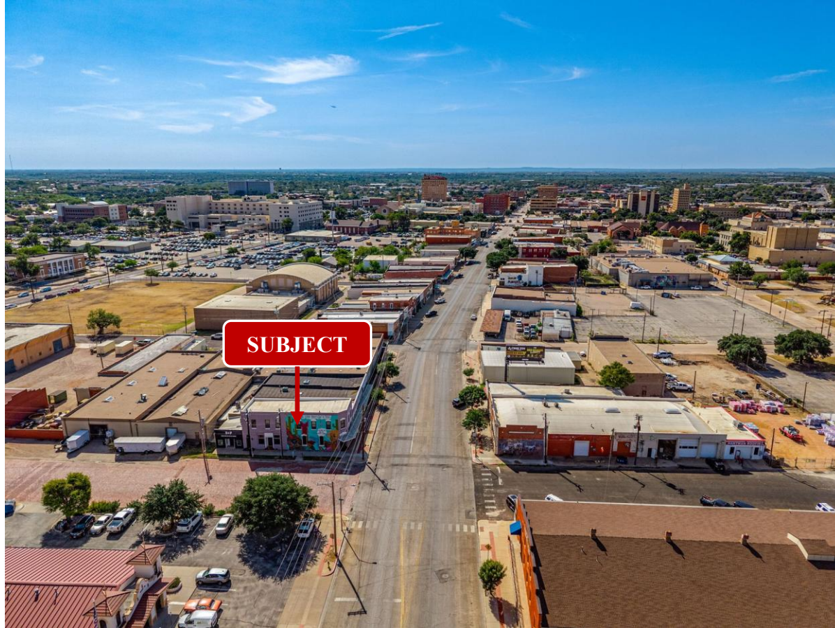
Looking south along N Chadbourne toward downtown
