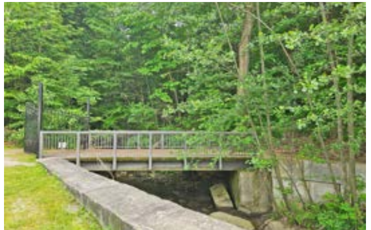
Bridge & Path Along Eastern End Of Site Near Baer Beach
