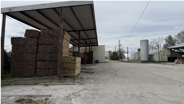
COVERED SHED, STACKED MATERIAL
