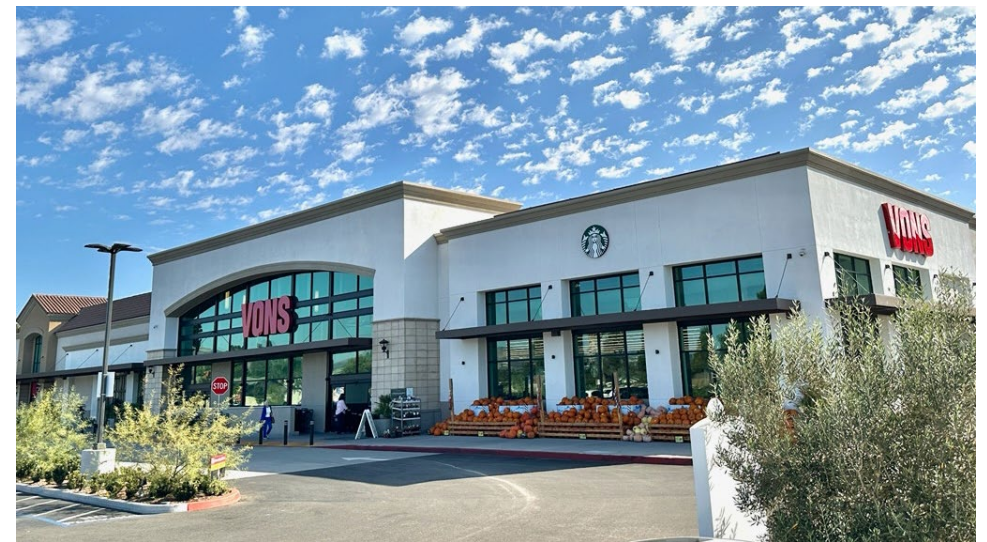
01 – Newly constructed 63,272 SF Vons
