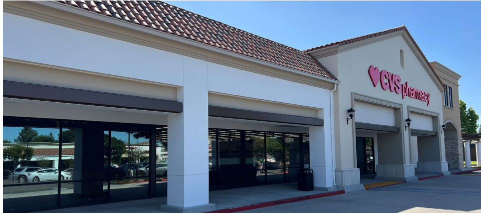
02 – 23,989 SF CVS with Full Façade Refresh
