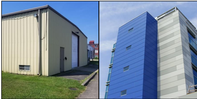
Figure 1327.C: On the left, metal sheeting which is prohibited. On the right, architectural metal panels.
