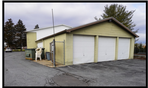
Garages and work shop
