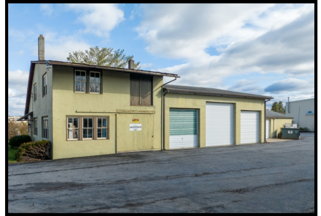
Garages and work shop
