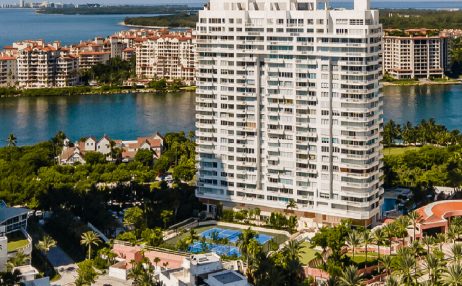
SOUTH POINTE TOWER
