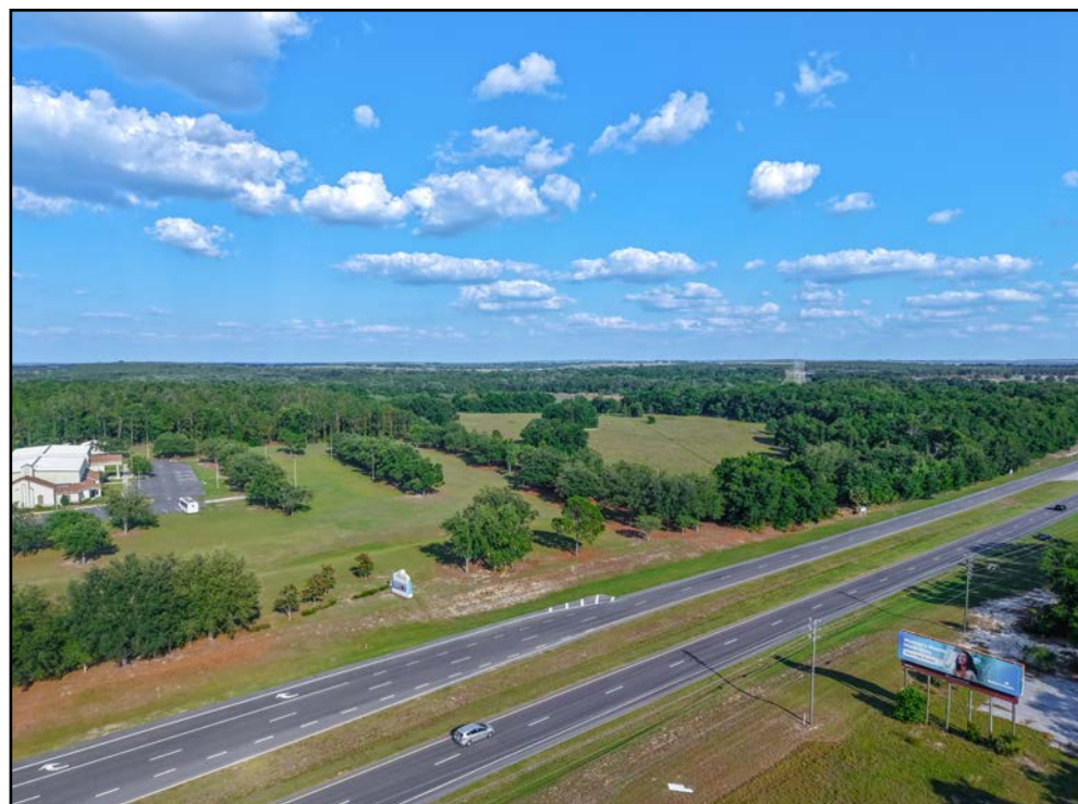
Looking from the northwest on US Highway 27
