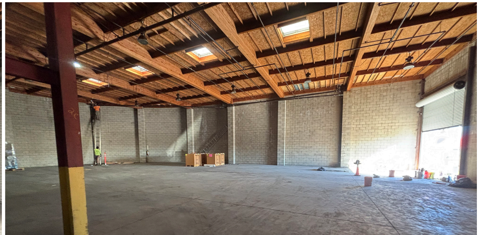
Concrete Block Addition (20' Clear)
