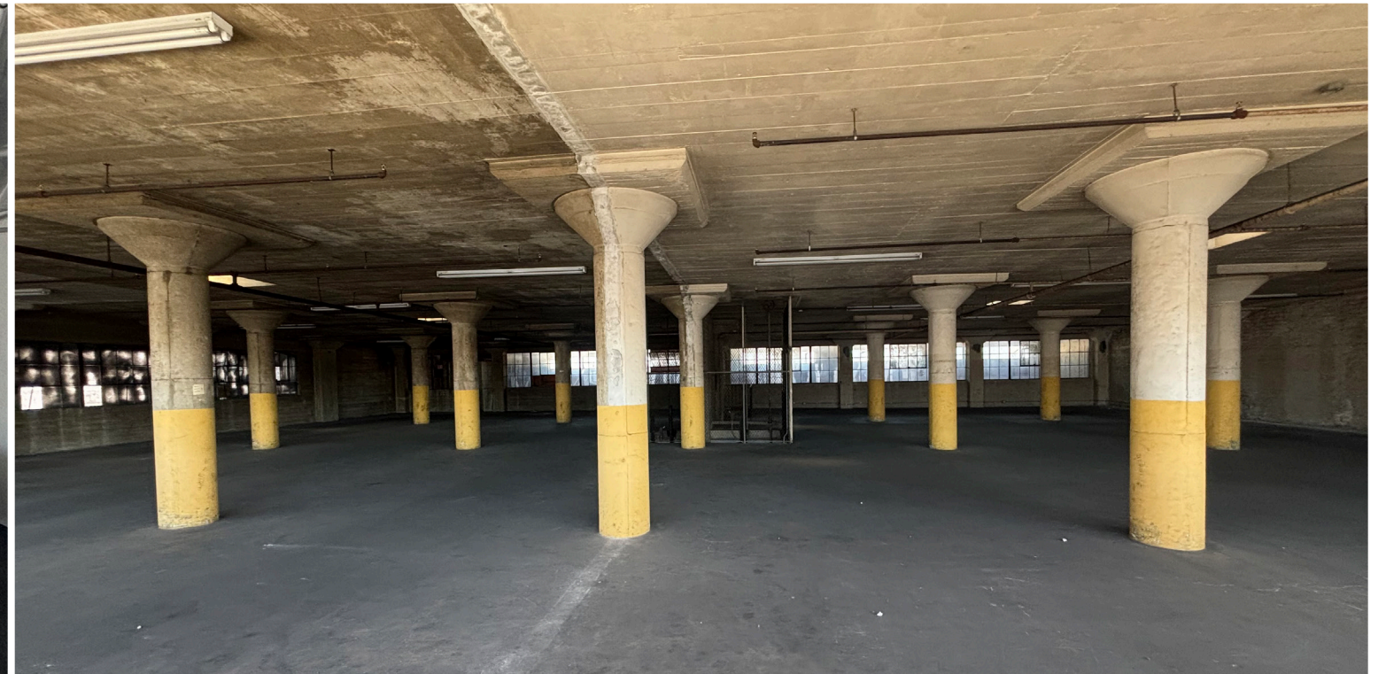
Third-Story Warehouse (12' Clear)
