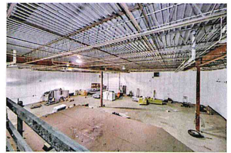
View of miscellaneous room
