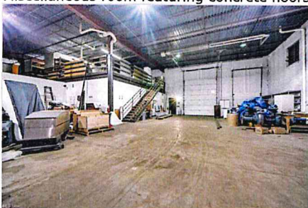
View of garage
