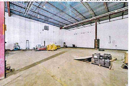
View of garage
