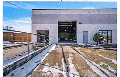
View of snow covered property entrance
