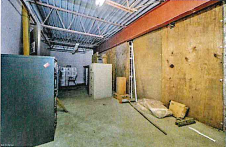
View of basement
