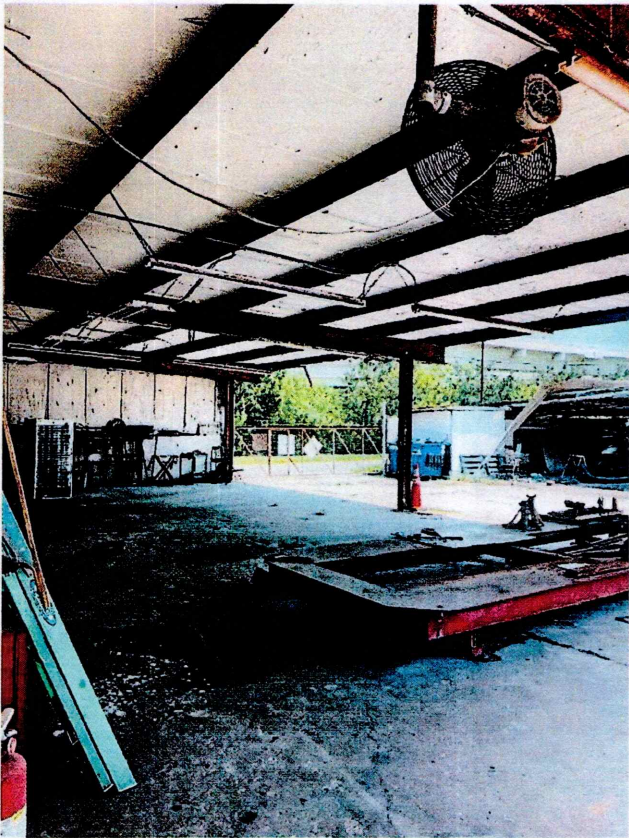
↑ Covered Work Area back of body shop
