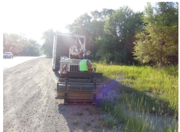
Photo 6: Preparing the drill rig. Photo taken by J. Hale 6/16/2014
