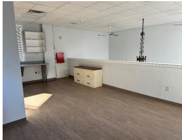
Suite A - Second Floor Office
