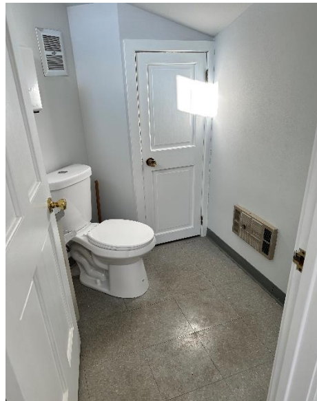
Suite A - Second Floor Bathroom
