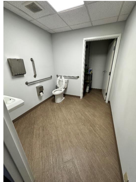
Suite A - ADA Bathroom on First Floor
