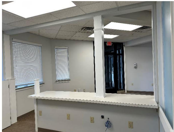
Suite B – Behind Counter
