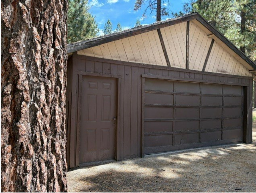
Moonridge Road - Garage
