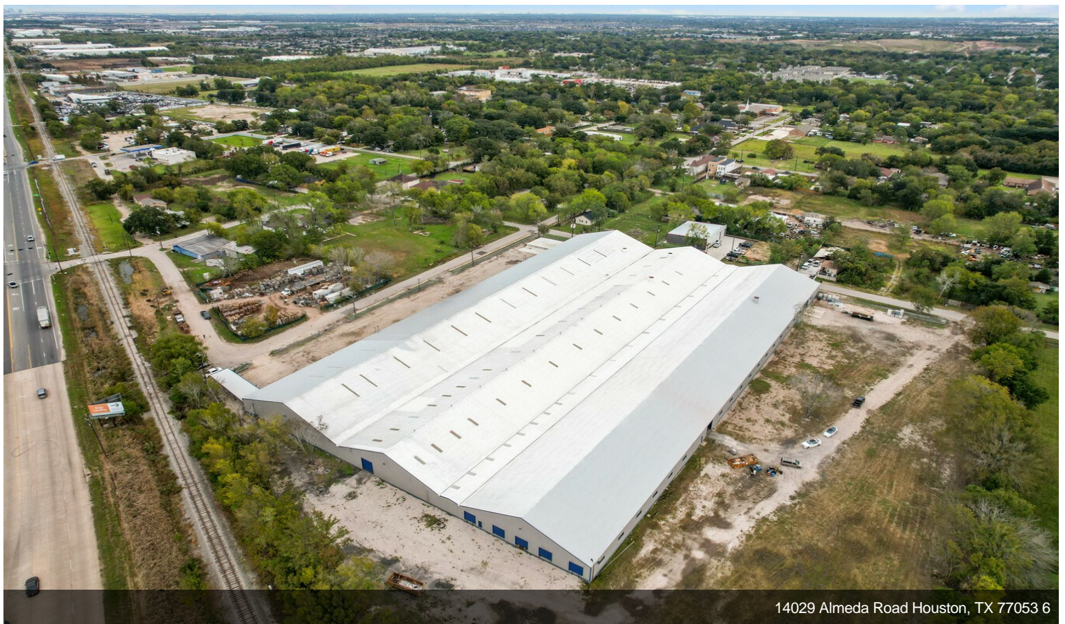
14029 Almeda Road Houston, TX 77053 29
