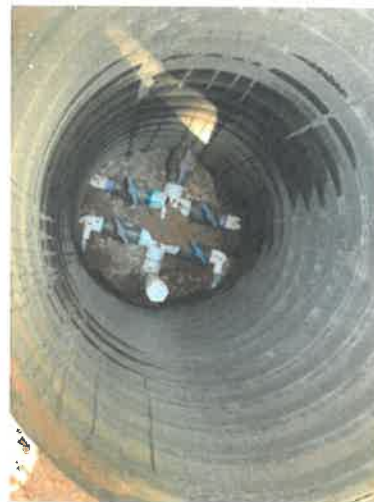
Figure 3: Flow Adjusting Ball Valves
