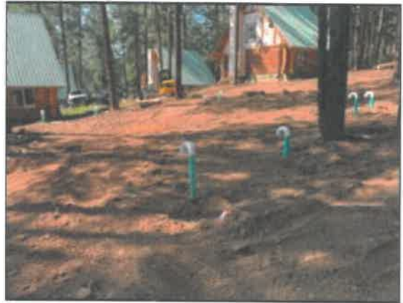
Figure 5: Final Site Grading Looking West
