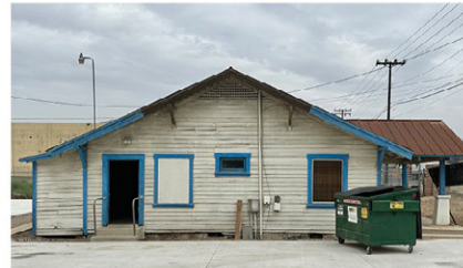
EX. BLDG. 2 - WEST ELEVATION
