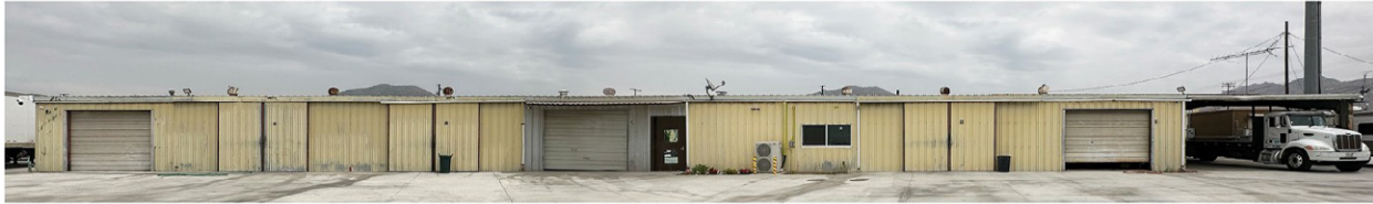
EX. BLDG. 1 - WEST ELEVATION
