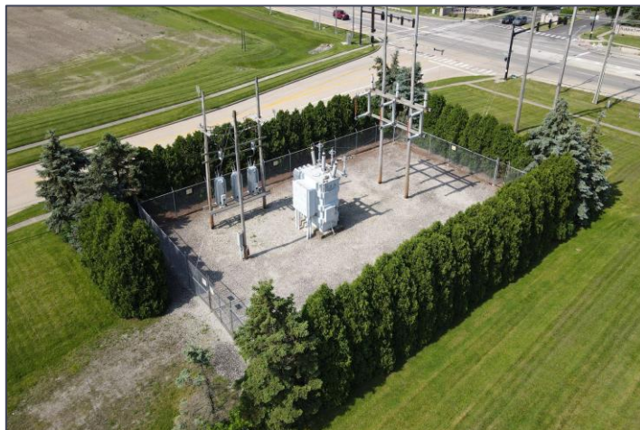
7.5/10.5 MVA 138 KVA Substation
