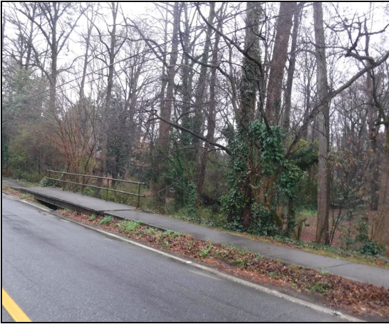
View of subject from Dresden Drive
