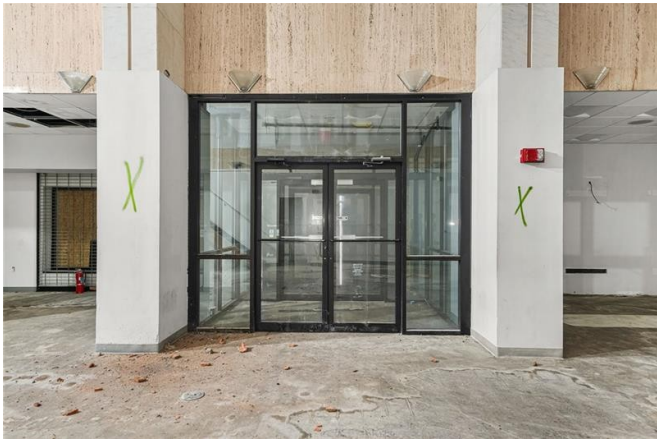
Commercial storefront entry — full-light glass doors with transom windows
