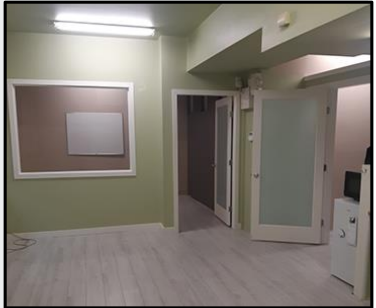
View from rear large office into private rear office
