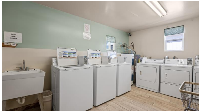
One of 2 Laundry facilities
