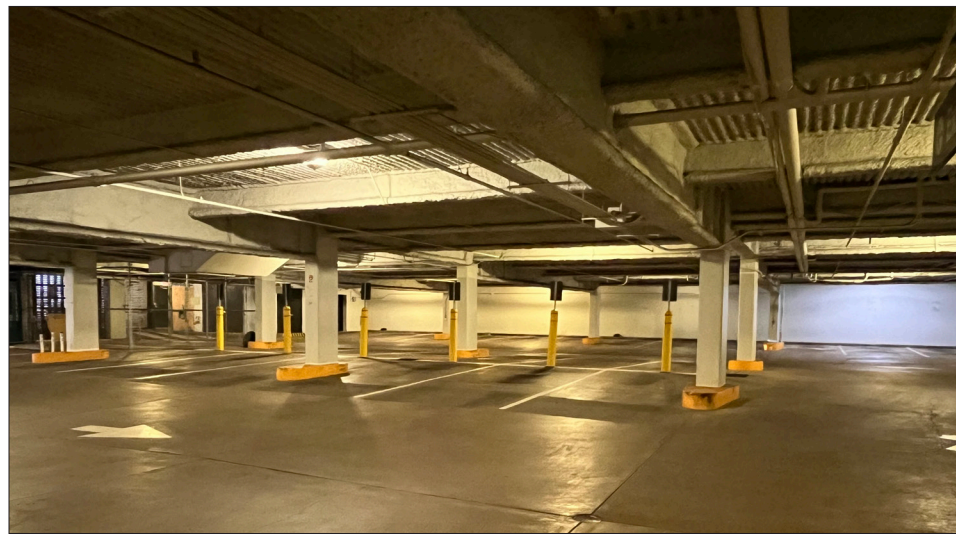
Secure 35 Car Parking Garage
