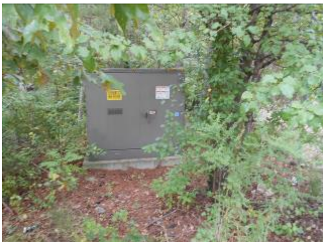
Pad-mounted, utility-owned transformer at the northern boundary of the subject property, east of the building.
