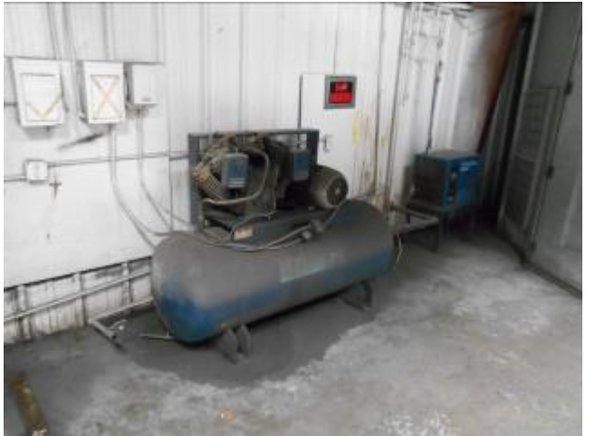
Compressor and air filter/dryer in southwestern corner of shop building. Oil staining observed on concrete floor.
