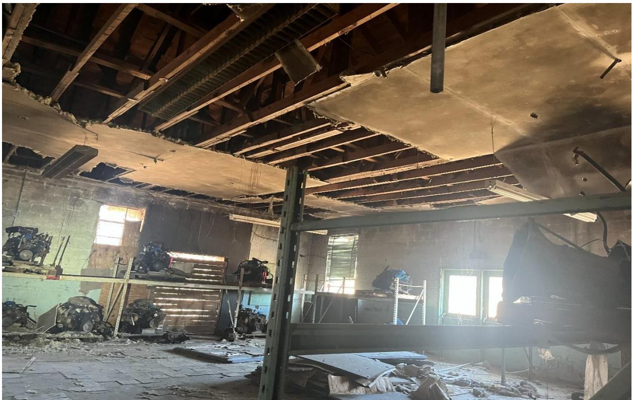
Interior of 12,078 SF Brick Building
