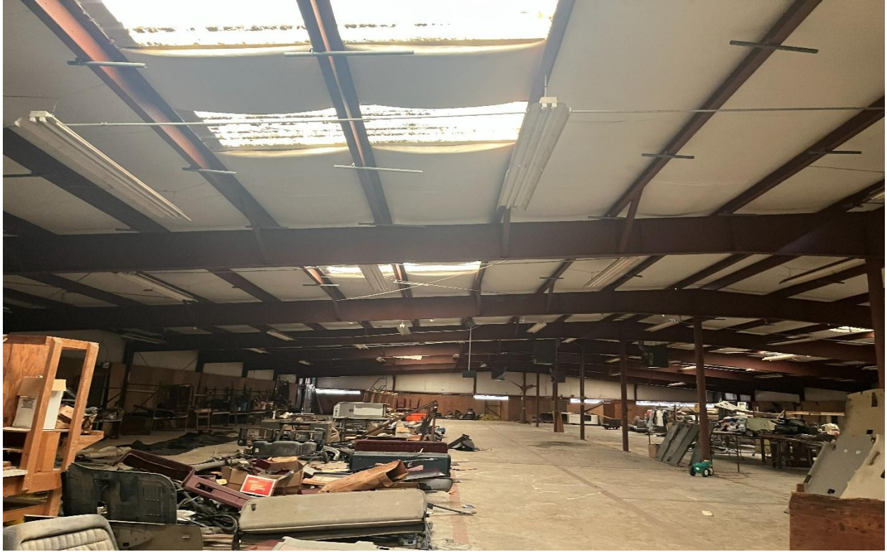
Interior of 18,000 SF Metal Building
