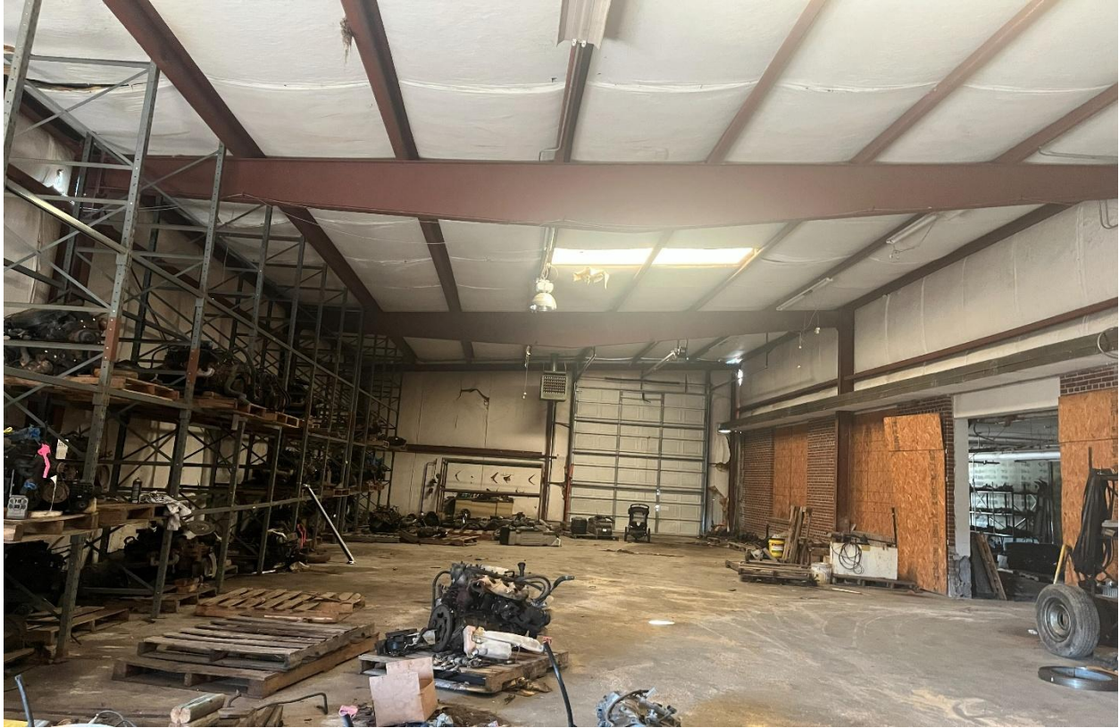
Interior of 5,736 SF Building
