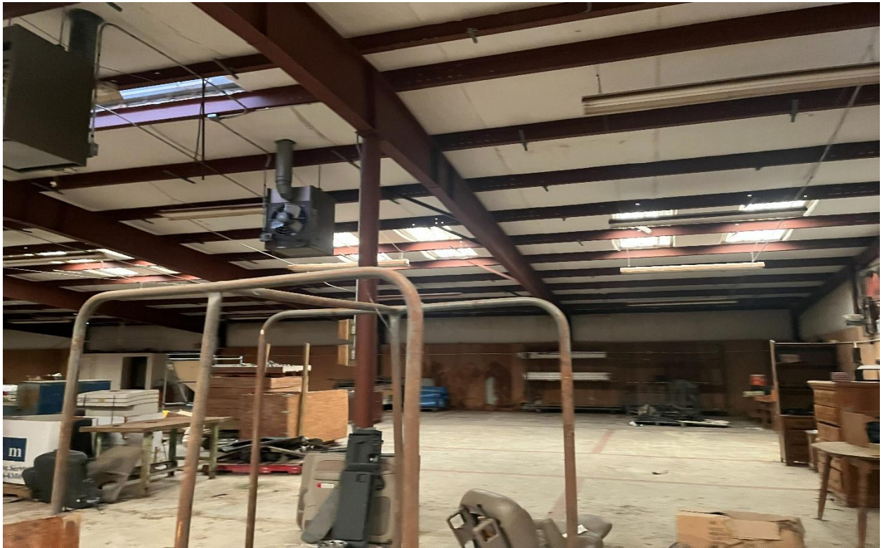
Interior of 18,000 SF Metal Building
