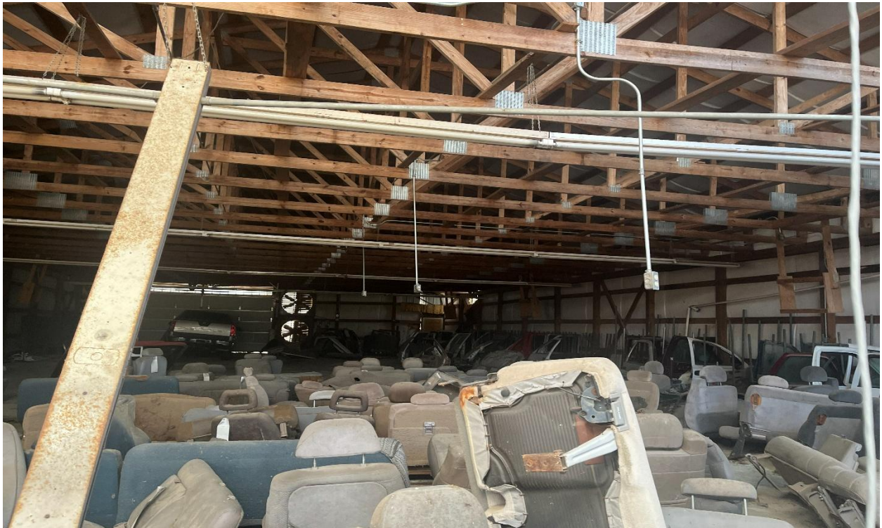
Interior of 4,998 SF Metal Building
