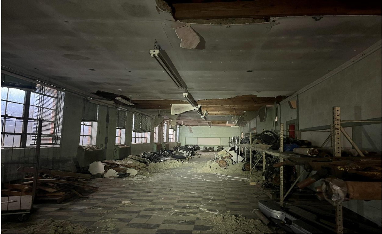
Interior of 12,078 SF Brick Building
