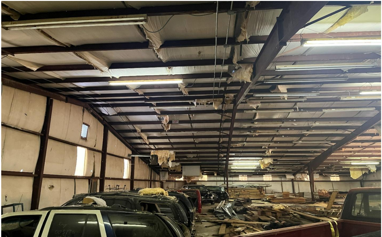
Interior of 10,500 SF Metal Building
