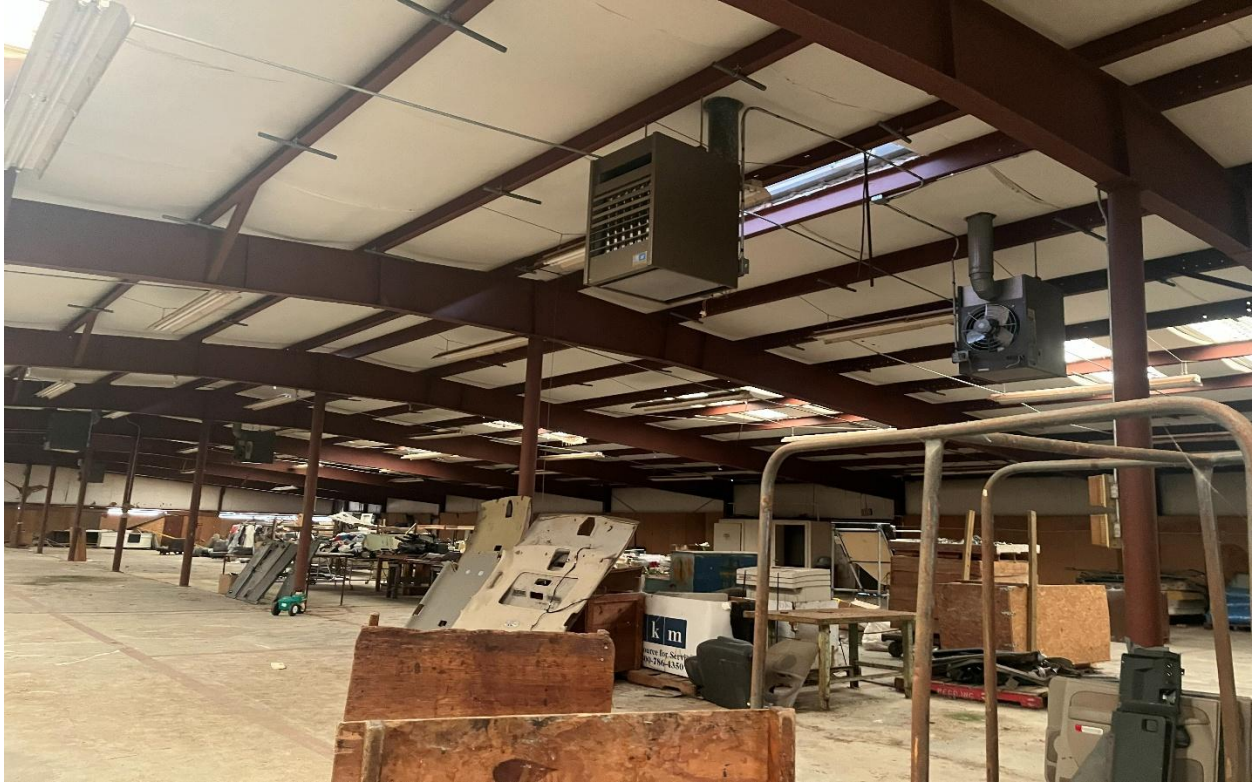
Interior of 18,000 SF Metal Building
