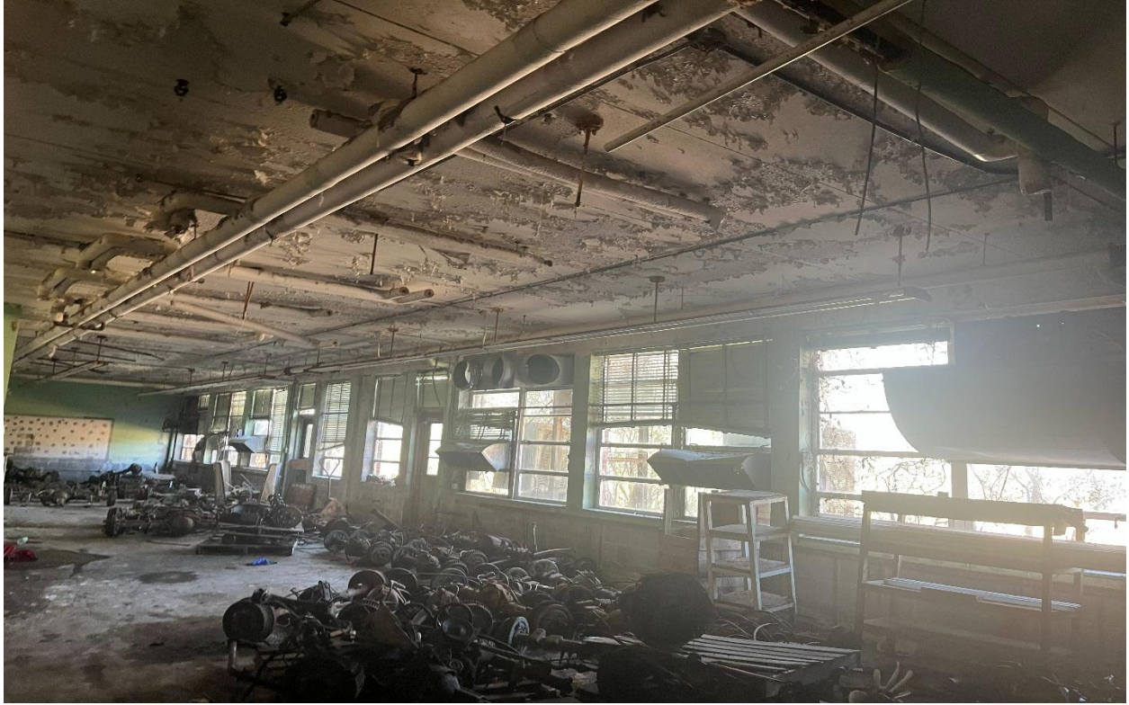
Interior of 6,874 SF Brick Building
