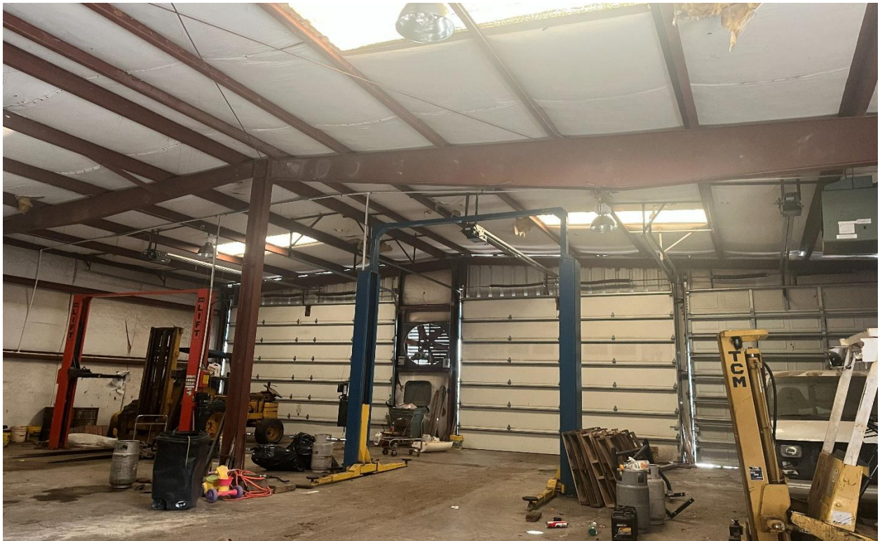
Interior of 5,736 SF Building
