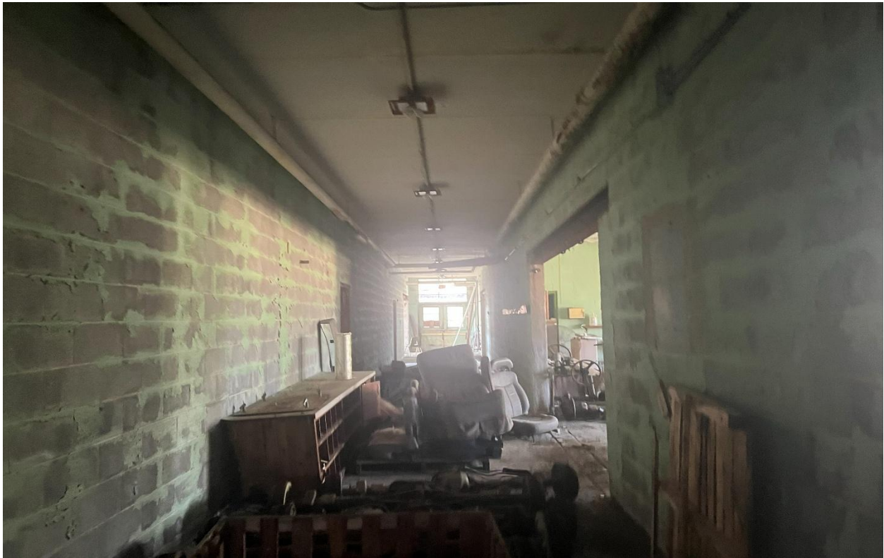
Interior of 6,874 SF Brick Building
