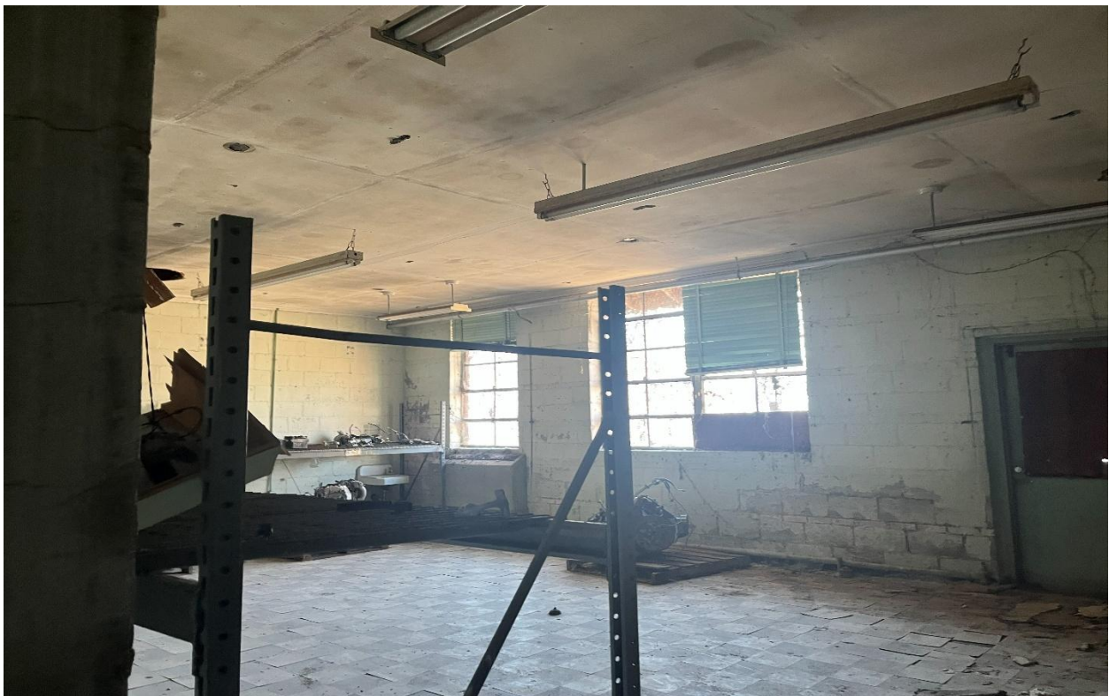
Interior of 12,078 SF Brick Building
