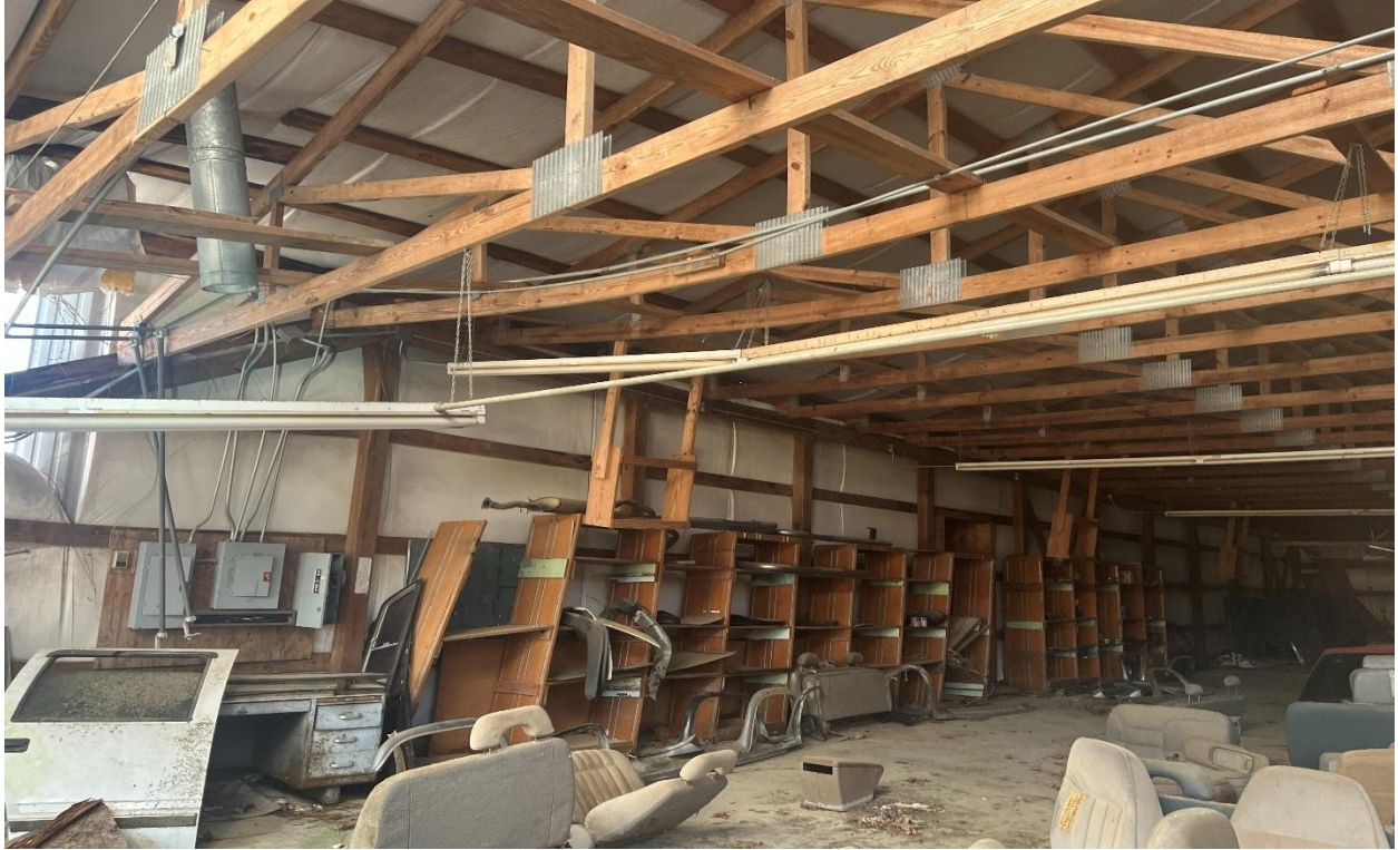
Interior of 4,998 SF Metal Building
