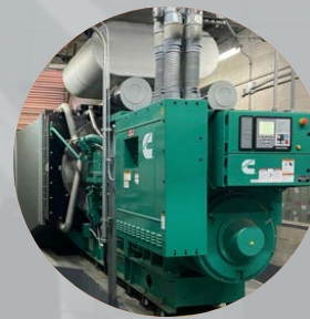
Cummins Generator 1000 KW with 2000 Gal Tank
