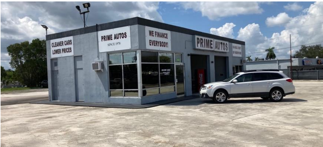
Photograph 2: View of the property looking towards the west.
