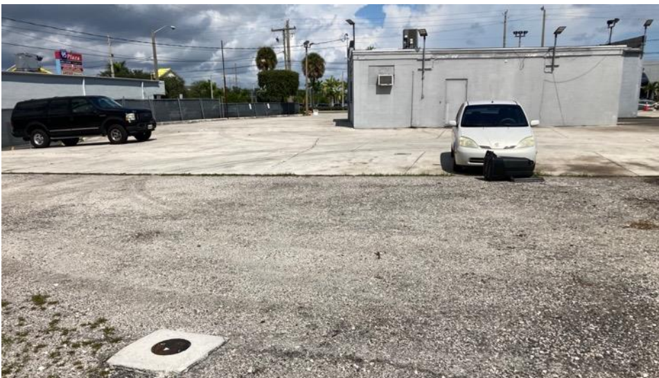
Photograph 3: View of the site, looking towards the north. Note the groundwater monitor well in the foreground.
