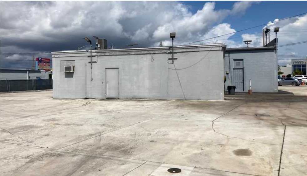
Photograph 4: View of the former underground tank area at the site looking towards the north.
