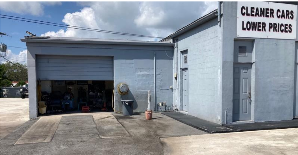
Photograph 5: View of the former repair shop area at the site.
