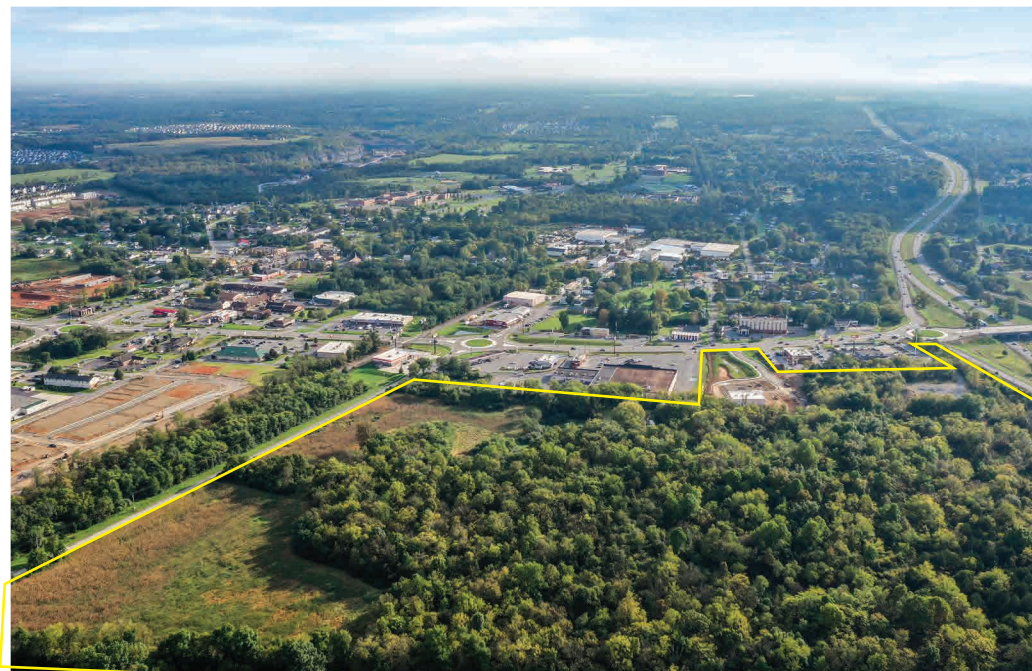
Aerial Facing South.
