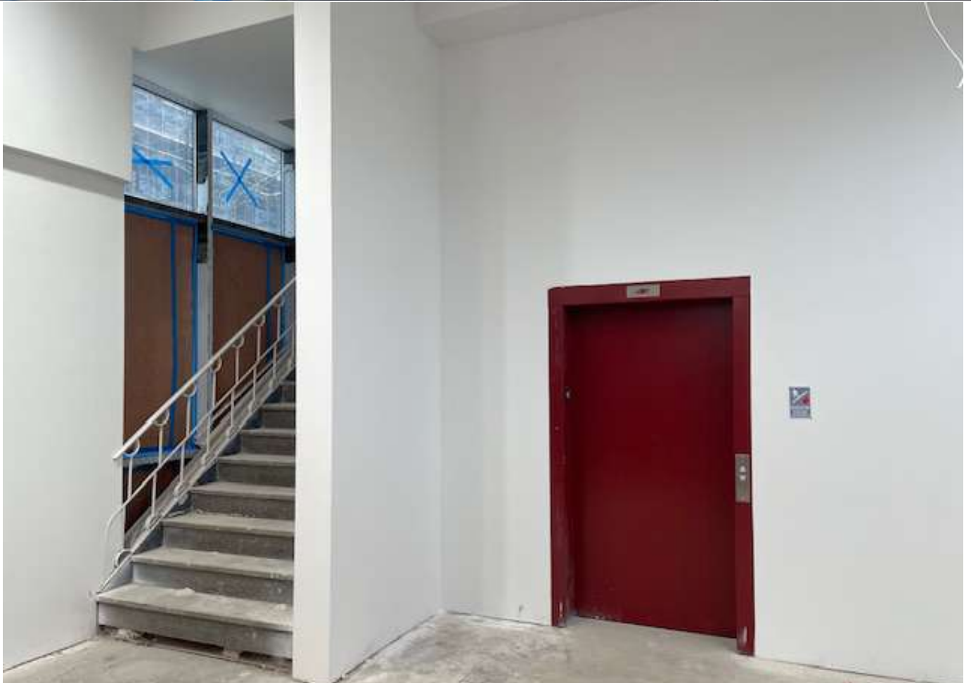
45TH STREET SIDE ELEVATOR
