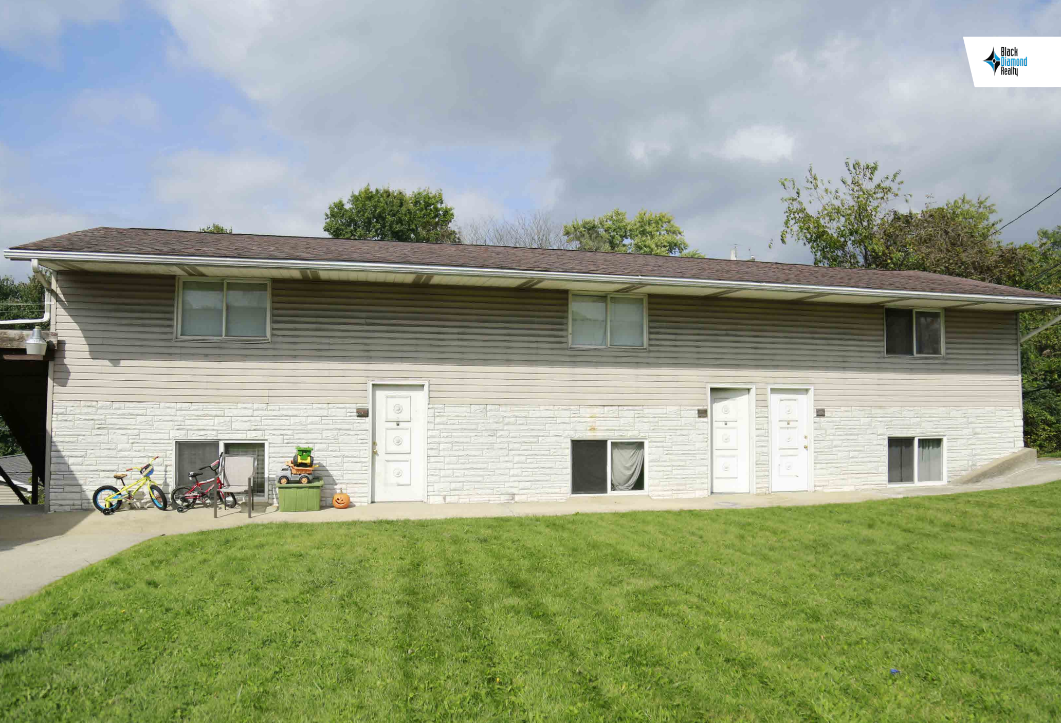
Building C - Exterior.
