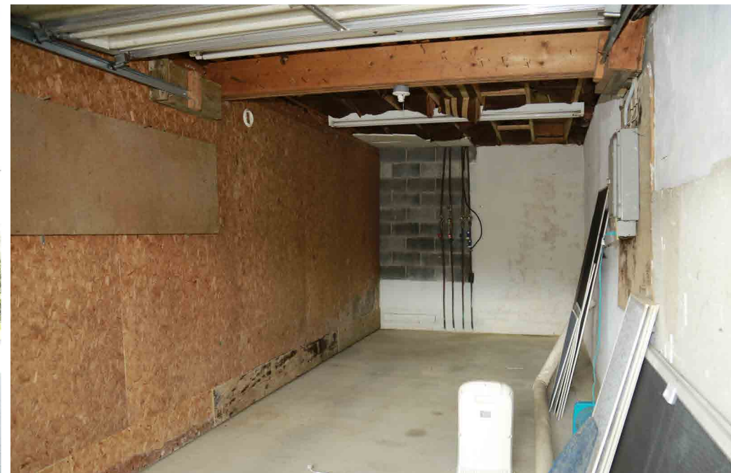
Building A Garage.
