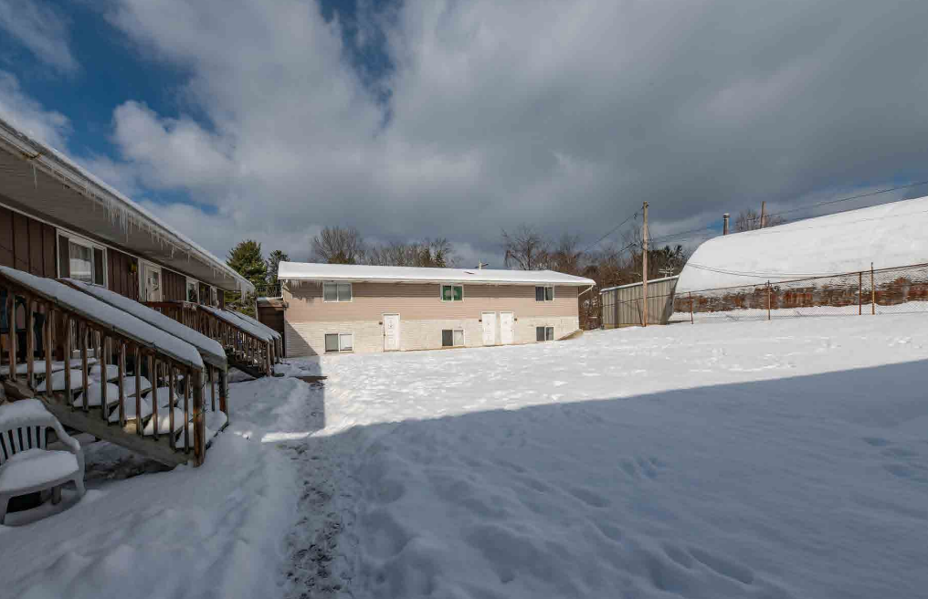
View of Building C from the Courtyard.
