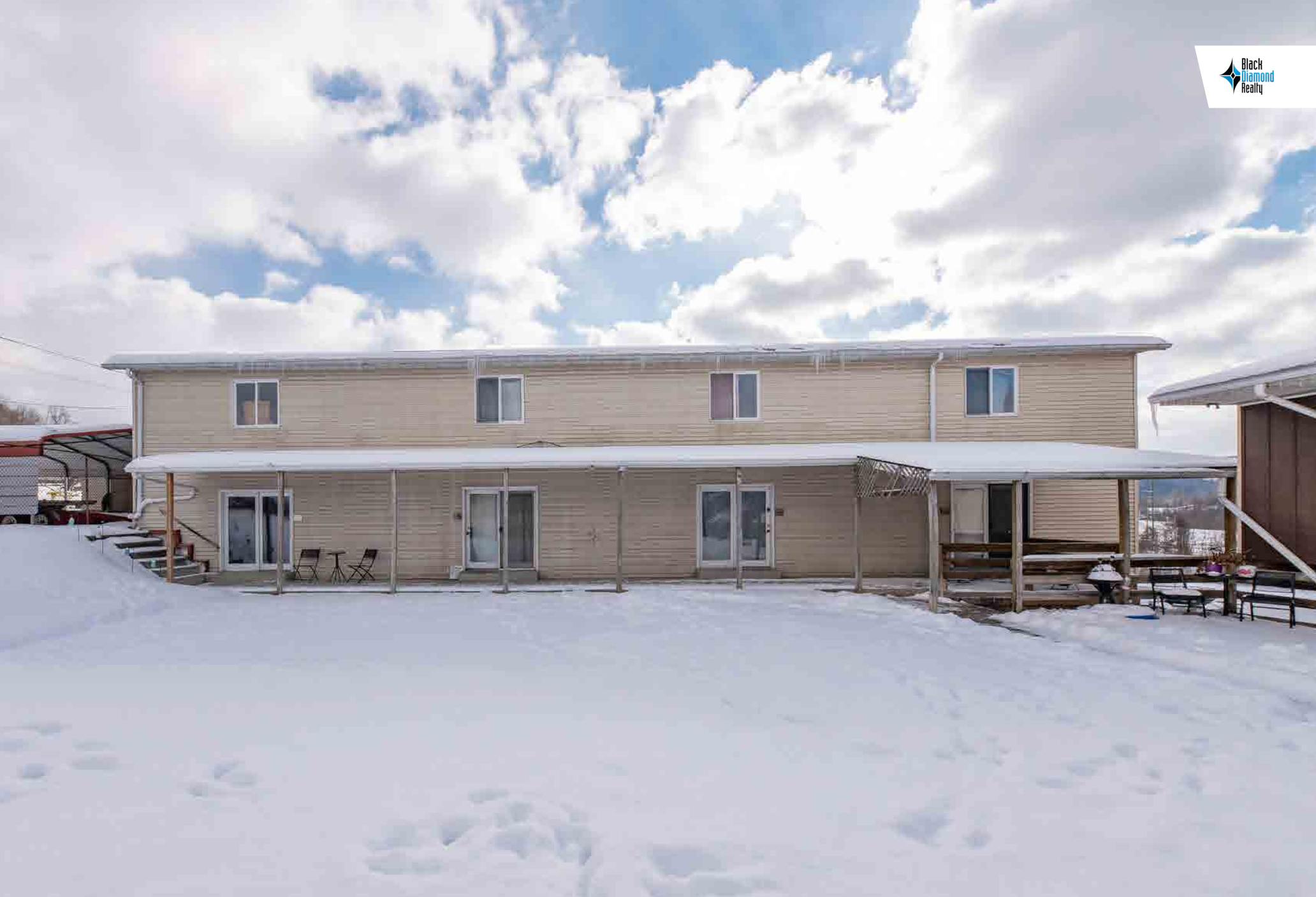
Building A - Exterior.
