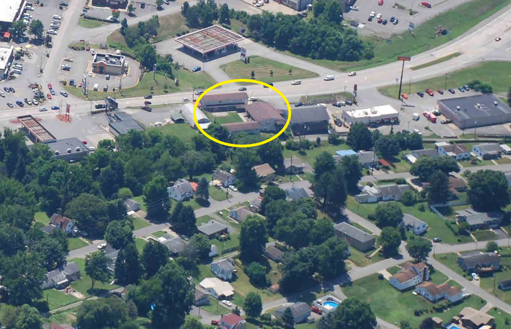
View of the Property Facing South.
