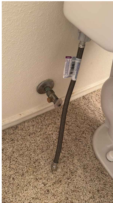
Upstairs Hallway Bathroom
