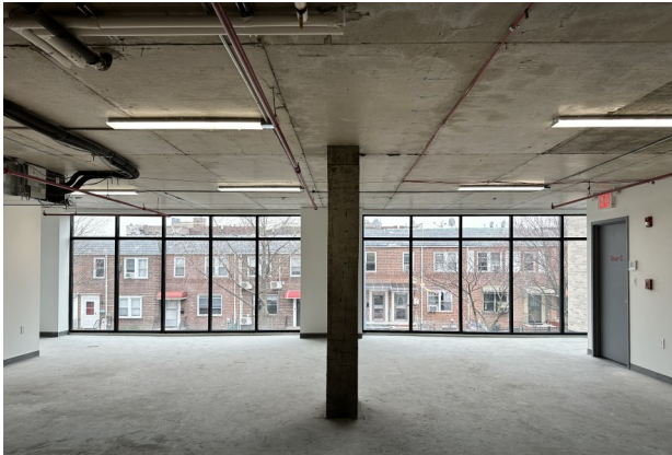
SECOND FLOOR MEDICAL OFFICE
