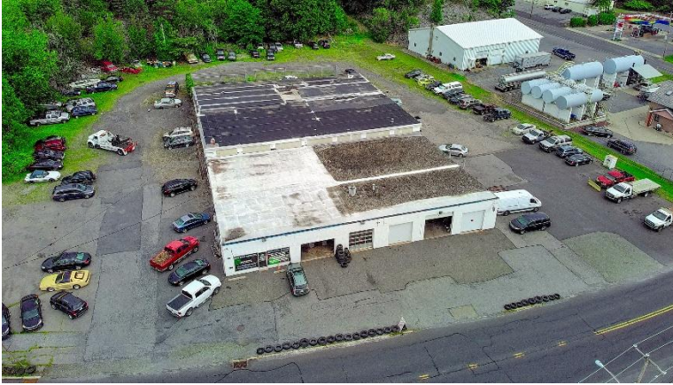
Front of building
