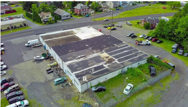
Rear / right side of building
