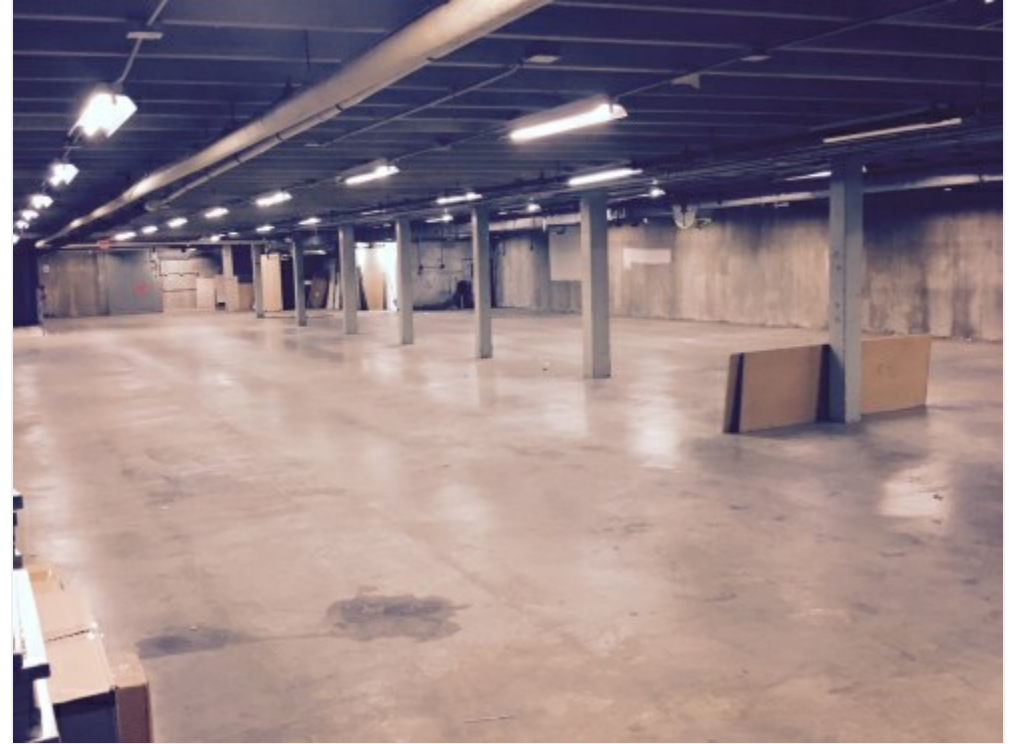
Basement - 6,600 s.f. - 8 ft ceiling
