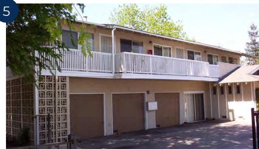
649 Nordale Avenue, San Jose, CA 95112
